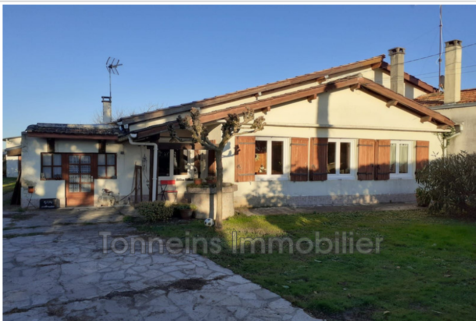
House 4031TI Saint-Pardoux-du-Breuil
